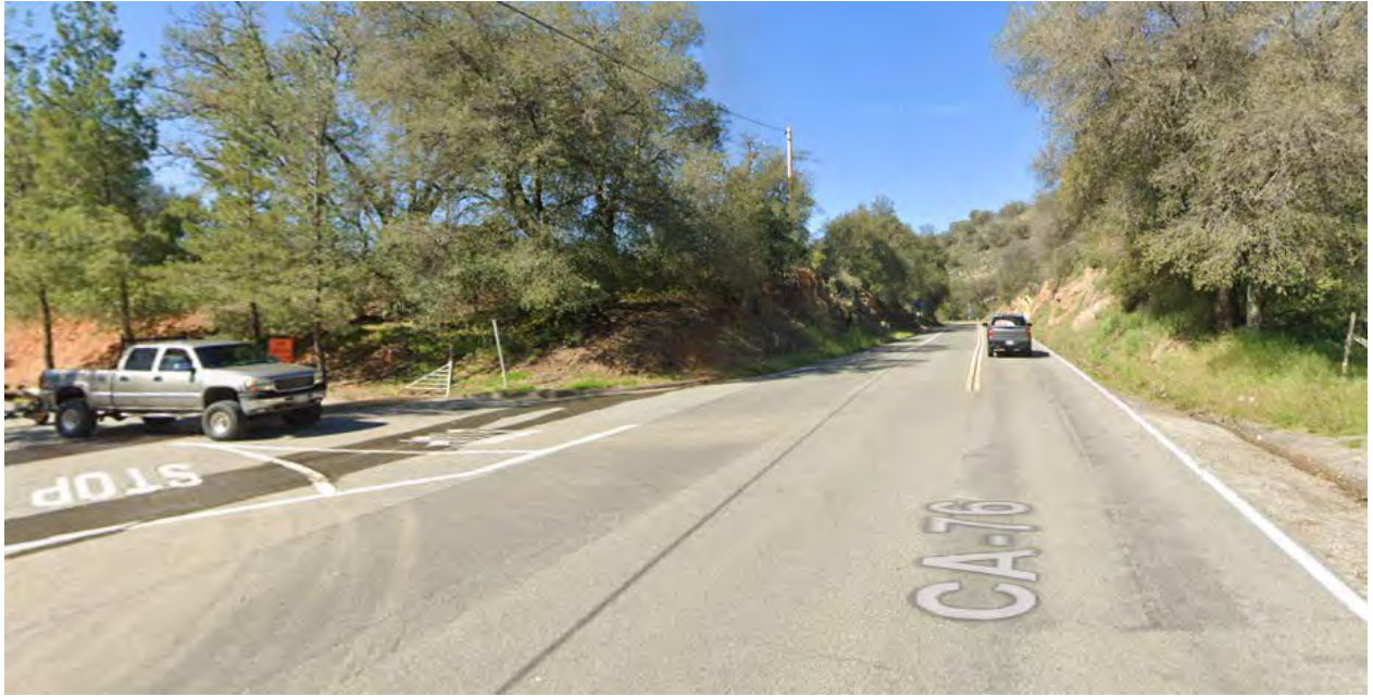
Figure 4-4: Northbound Traffic View on Sengme Oaks Road Looking West
