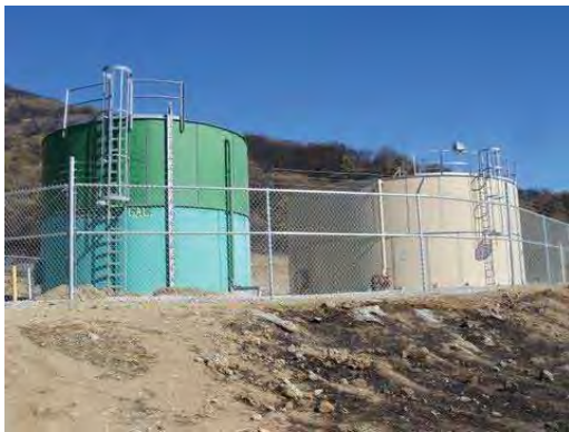
Picture 15 Water Towers
