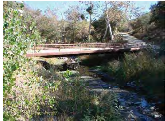
Picture 17 Bridge over the River at the Campground
